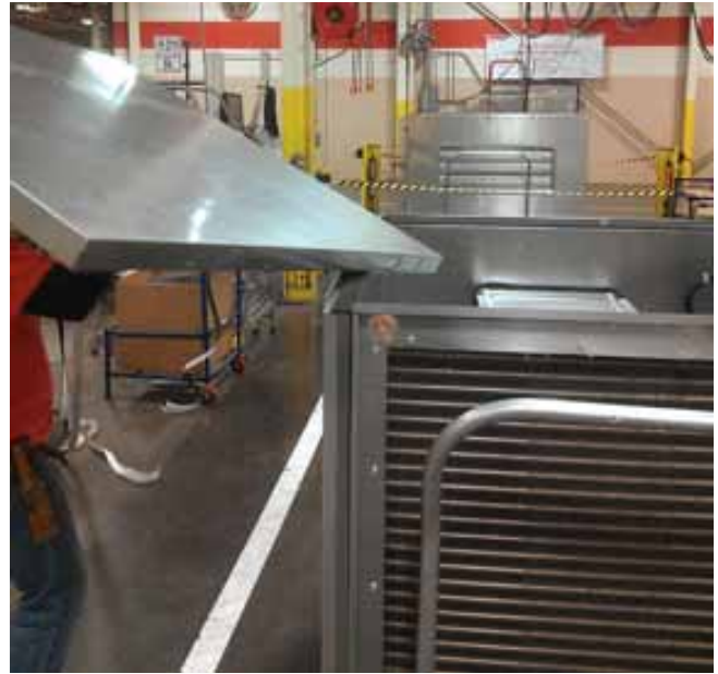
Figure 8. Lift the roof panel off
