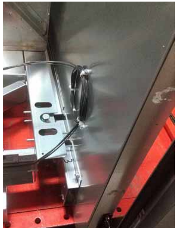
Figure 19. Remove screw ties holding high voltage wiring harness
