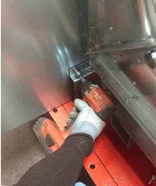
Figure 20. Support walls to prevent falling
