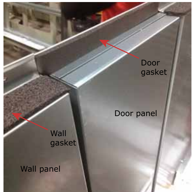
Figure 9. Replace gasket if needed
